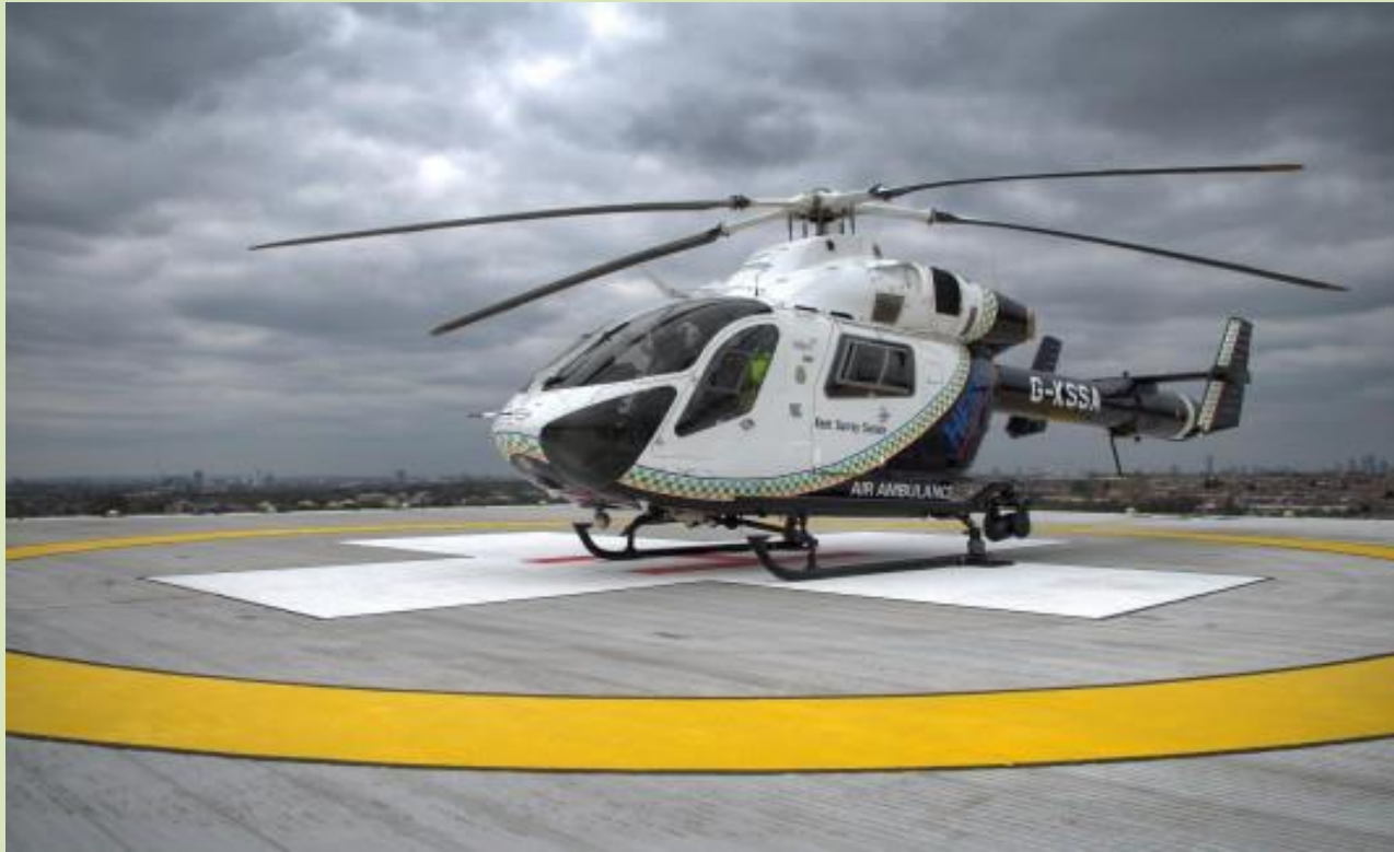
Helipad near DG & ADG quarters
